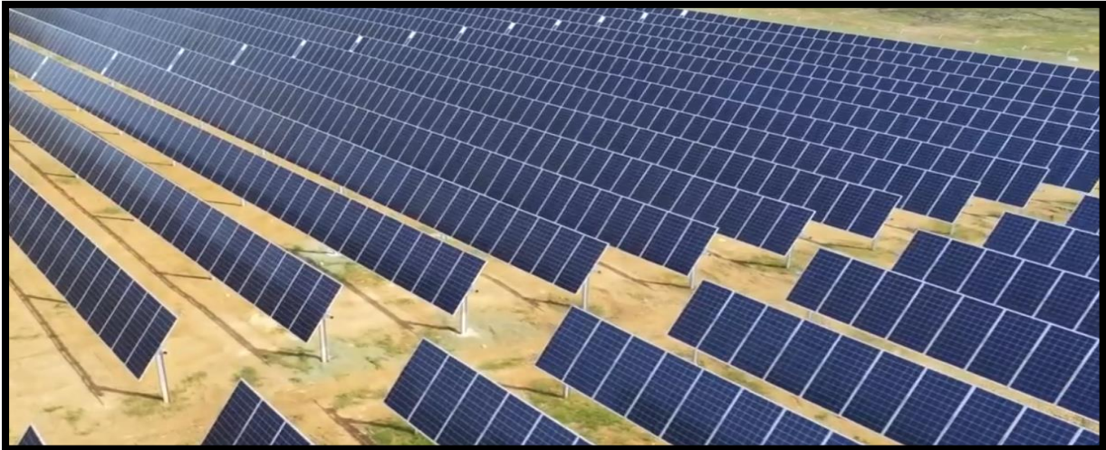
Fig. 4: Trackers with backtracking arrangement
