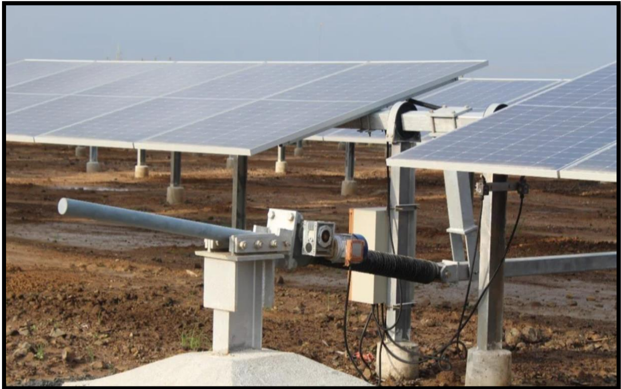
Fig.5: A Gang-type tracking system with an actuator stroke-rod
