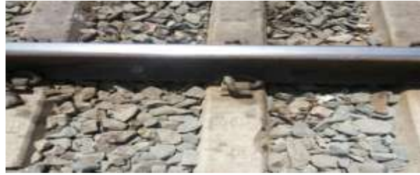
Fig No: 1.1 Clamps in Southern Railway Track
