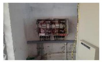
Fig.2. Solar array junction box
