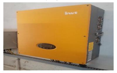
Fig.3. Solar grid inverter
