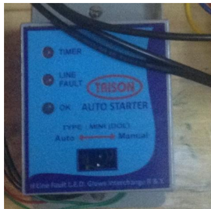
Fig 2.4 Relay for operate in wrong phase sequence.
