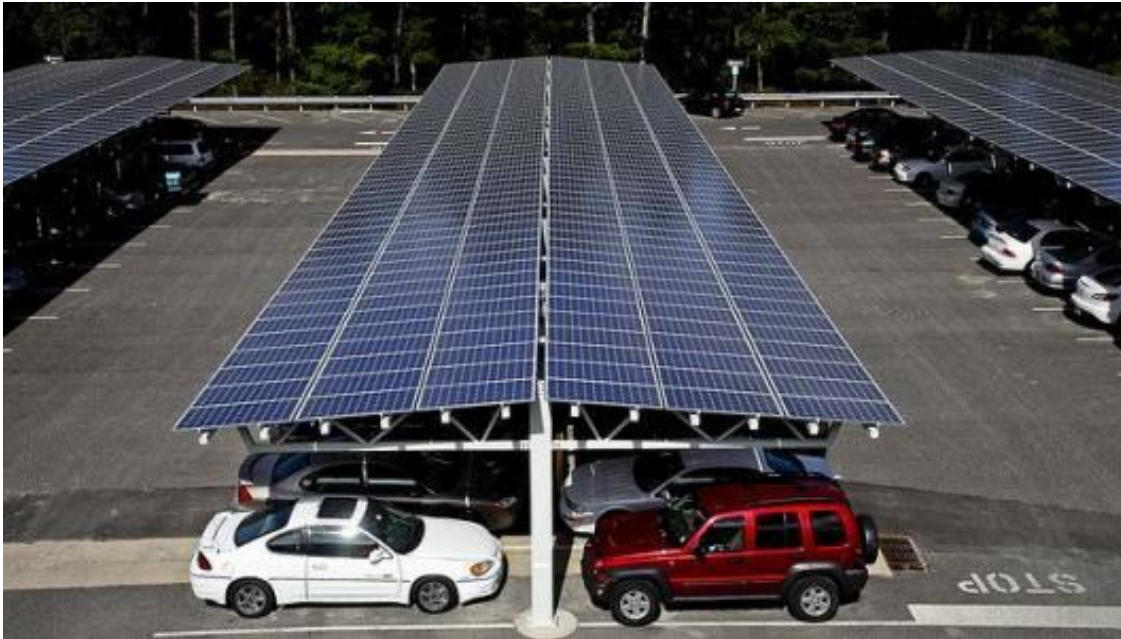
Fig.(3)Electricity generation by solar (By placing solar panels on roof of parking )
